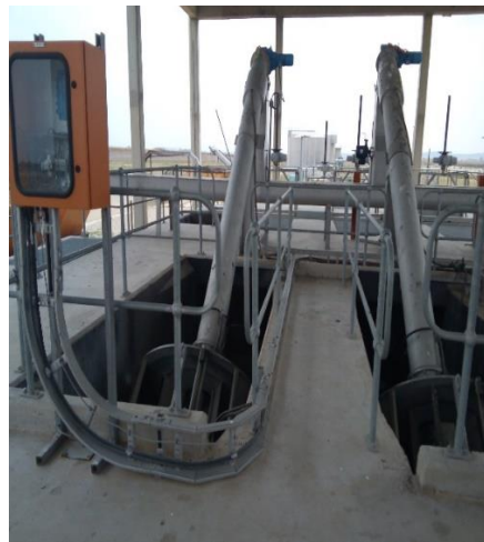
Figure 3.11 Rotary drum screens at the NEWTW (Author's own, 2023)
