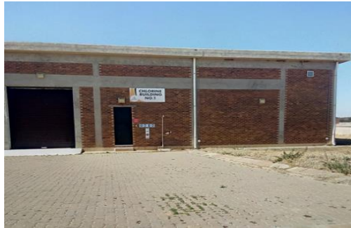
Figure 3.18 Chlorination room at the NEWTW (Author's own, 2023)
