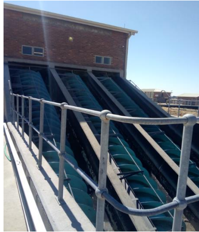
Figure 3.9 Screw pumps at the NEWTW (Author's own, 2023)
