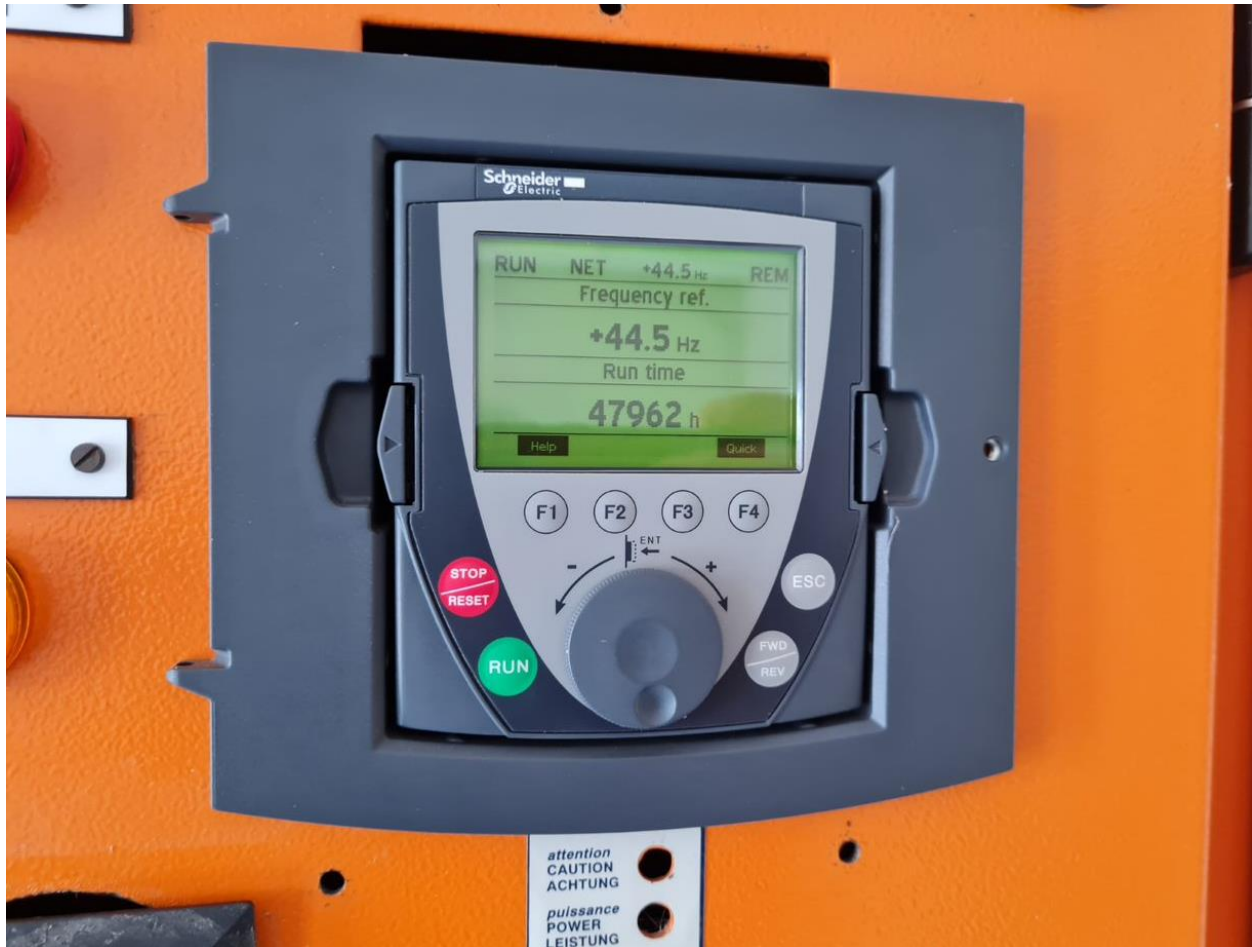
Figure 4.3: VFD pump control
