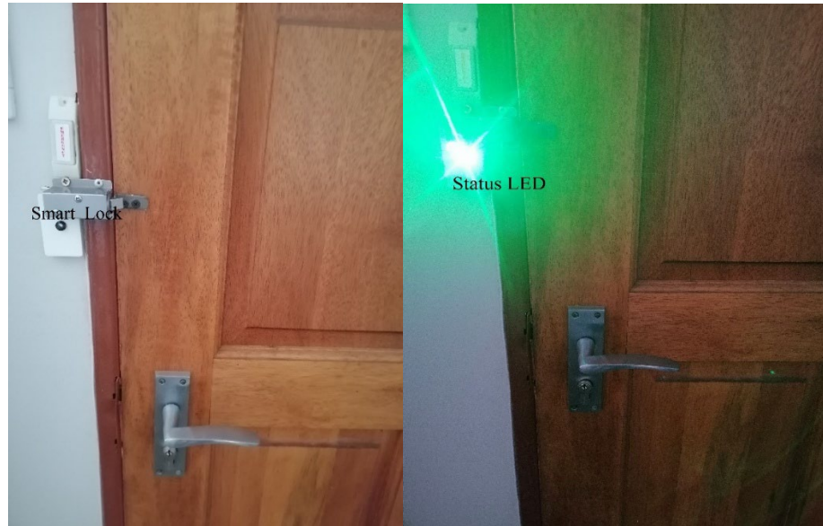
Figure 15: Main Access Door Alarm Status
