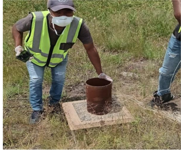
B – The open borehole outside the landfill which has a pronounced collar
