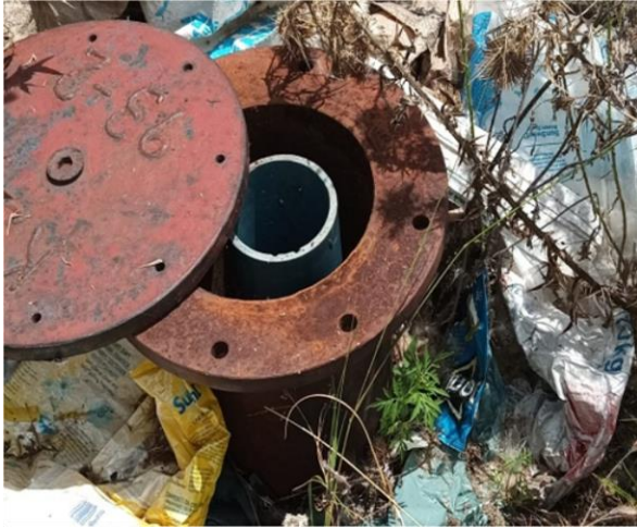
A – A capped borehole at the landfill site surrounded by plastic waste
