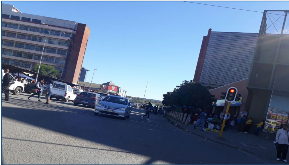
Figure 3.15 Facilities for traffic management (signalling and pedestrian crossings) at the intersections in Mthatha
