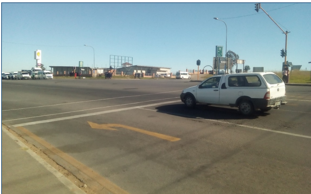
Figure 3.16 Facilities for traffic management (pavement markings and lane delineations) at the intersections in Mthatha
