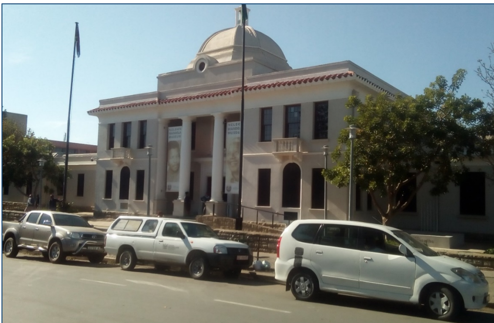
Figure 3.18 Road markings indicating on-street parking spaces and lane delineation on Mthatha's roads. Source: Author's own (2019)
