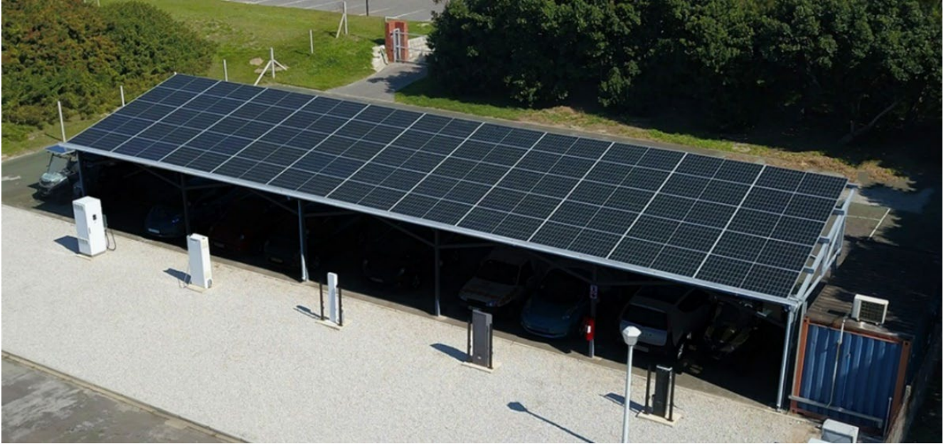
Figure 3.8: Current design of the EVCS at NMU (Uyilo) [150]
