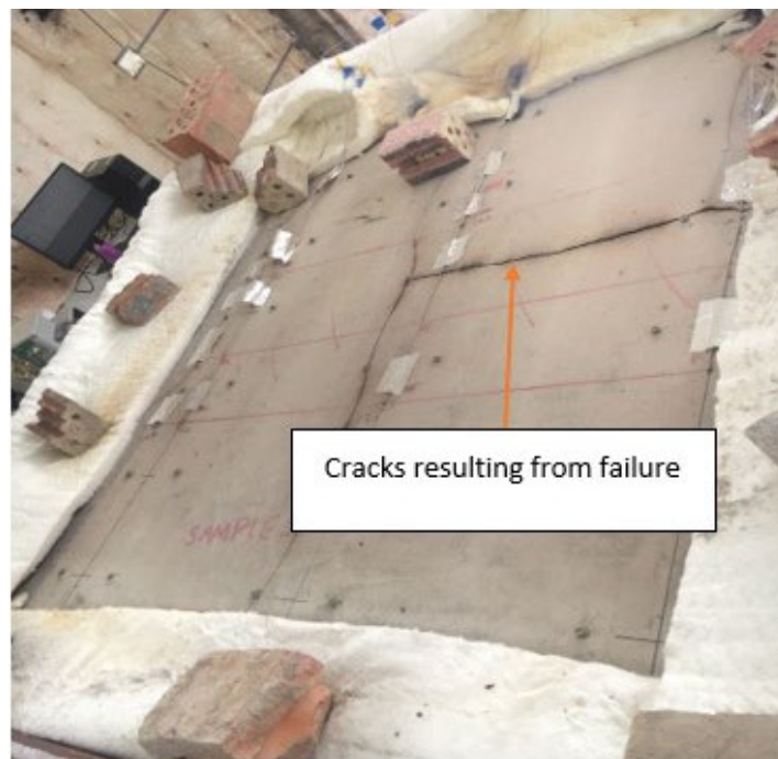
Figure 45. Cracks showing on the unexposed FCB at failure
