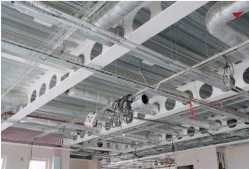
Figure 11. Cellular beams with service holes in them
