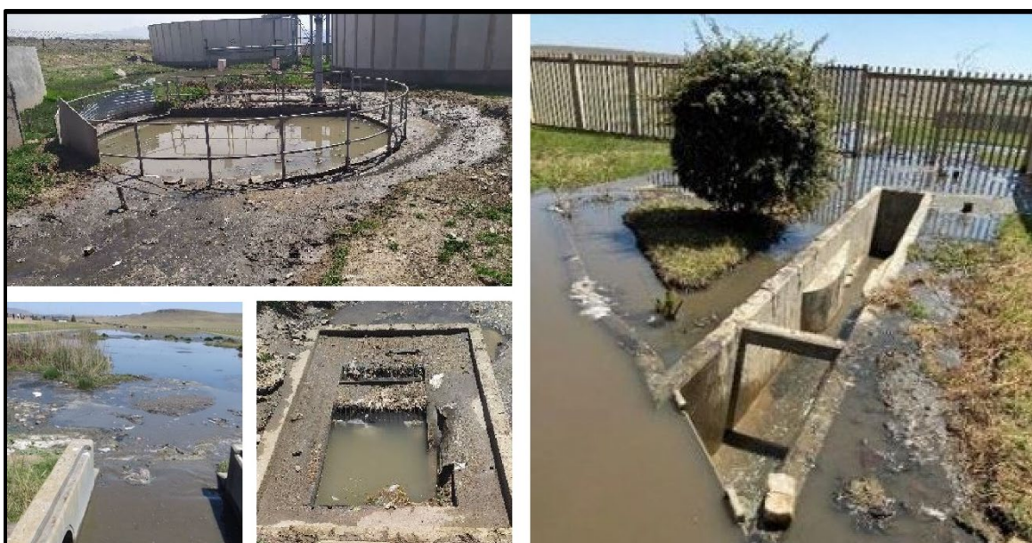
Figure 2.9: Infrastructural failure of WWTPs in the FS province (DWS, 2022b)
