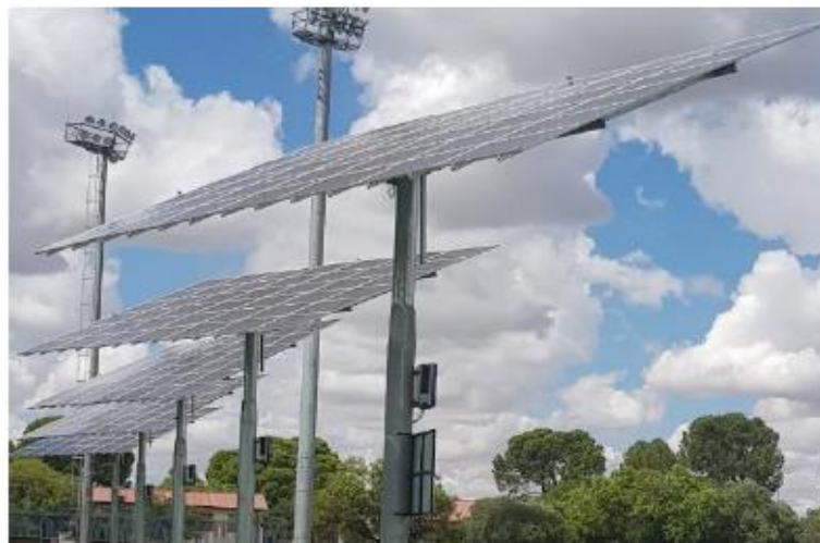
Figure 3.1: Dual-axis PV tracking systems installed on the Central University of Technology, Free State's (CUT) premises [117]
