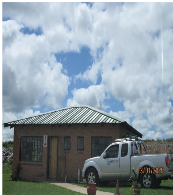
Annexure 1.14: A functional landfill site office with ablution facility, running water and electricity in Bethlehem
