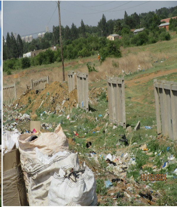
Annexure 1.8: Precast concrete panel fencing vandalised in the Viljoenskroon landfill site
