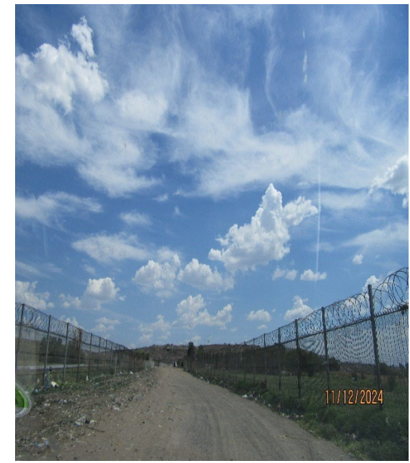
Annexure 1.10: Diamond link wire mesh with razor wire topping, well-maintained in the Sasolburg landfill site
