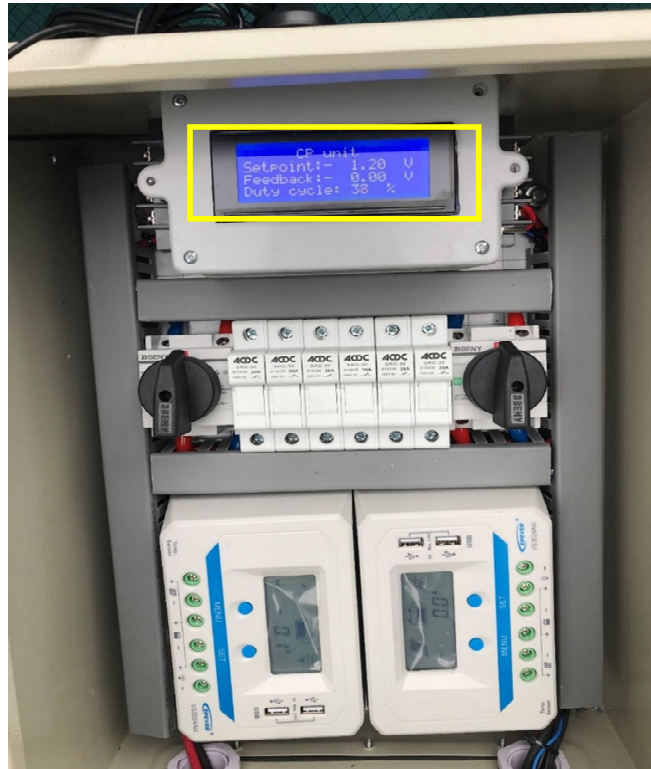
Figure 5.9: CPU site testing with 38% duty cycle
