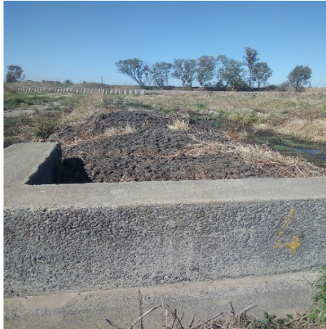
Figure 3.5 Sludge drying beds at the BWTW (Author's own, 2023)
