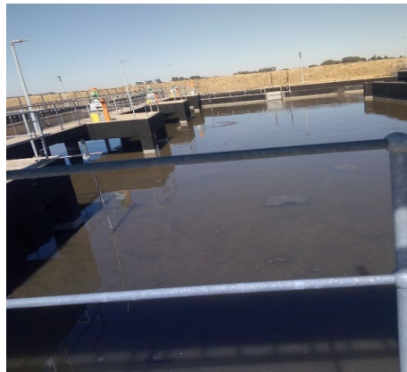
Figure 3.14 Grit settling tank at the NEWTW (Author's own, 2023)
