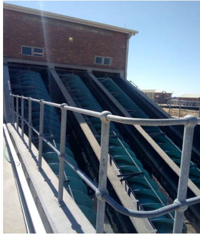
Figure 3.9 Screw pumps at the NEWTW (Author's own, 2023)
