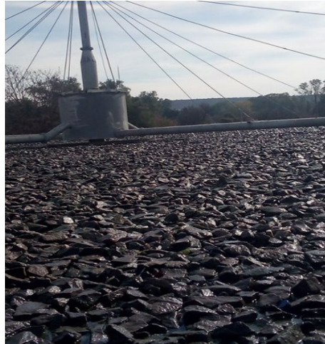
Figure 3.6 Trickling filter at the BWTW (Author's own, 2023)
