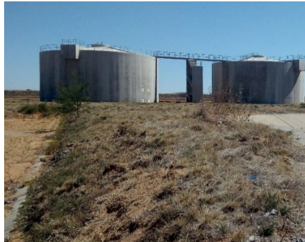
Figure 3.16 Digester tanks at the NEWTW (Author's own, 2023)
