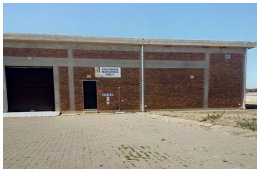
Figure 3.18 Chlorination room at the NEWTW (Author's own, 2023)
