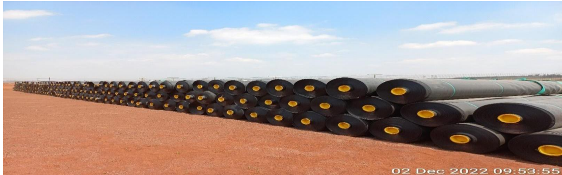
Figure 3.2: High-density polyethylene material for lining the landfill site
