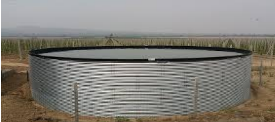
Figure 6.3: Leachate holding tank
