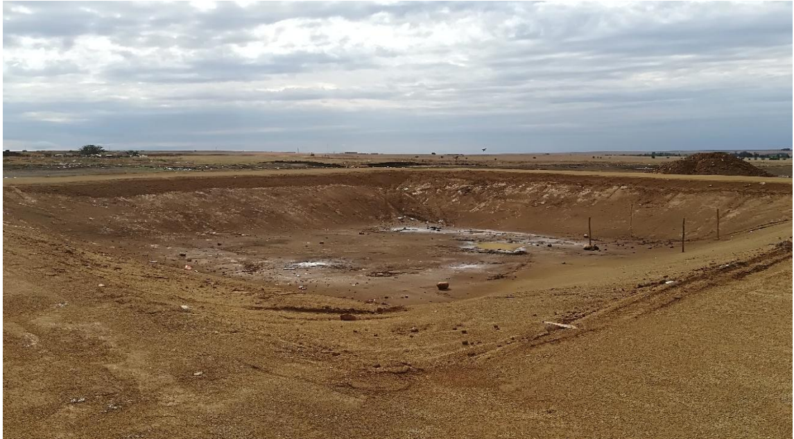
Figure 3.1: Construction of the leachate collection basin in the Free State province landfill site
