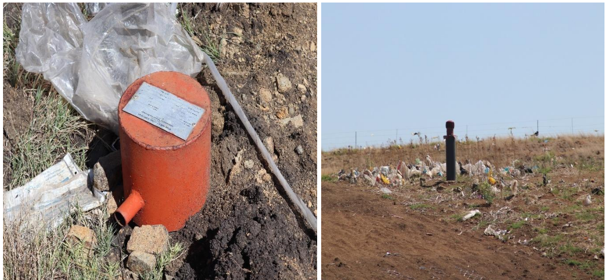
Figure 5.41: Boreholes up gradient and down gradient of a landfill site in the Free State province
