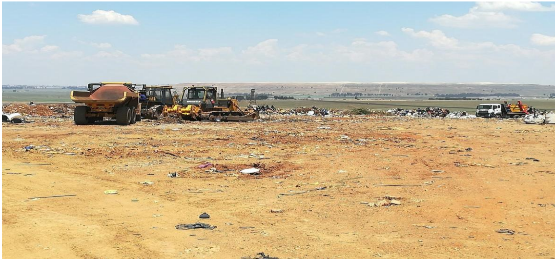
Figure 3.6 Tipper truck, compactor and a bulldozer at the Gauteng landfill site. Source: Noe, 2018
