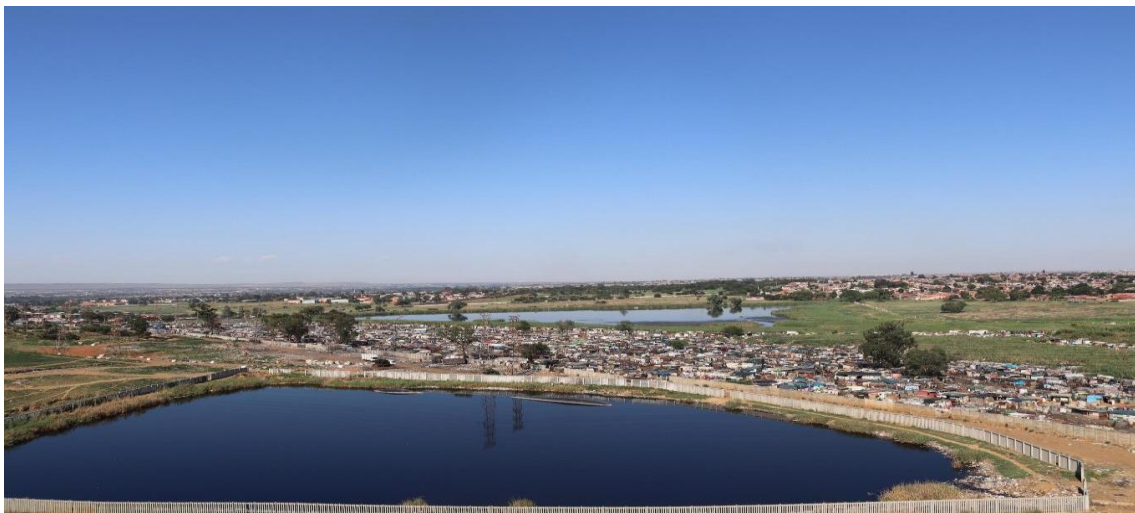
Figure 5.46: Leachate collection system at a Gauteng province landfill site. Source: Noe, 2018
