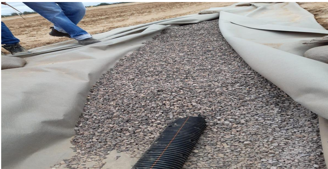
Figure 3.4: Drainage pipe covered with stones and wrapped with the geotextile Source: Noe, 2021
