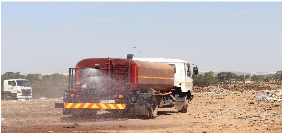
Figure 3.5: Dust suppression applied after the compaction of waste at the Gauteng landfill site.
