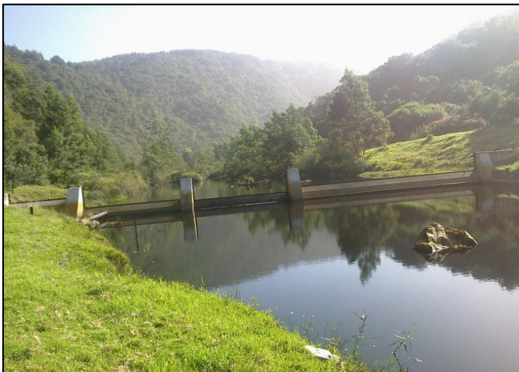
Figure 5.22: Gauging weir K2H002 in the Groot Brak River
