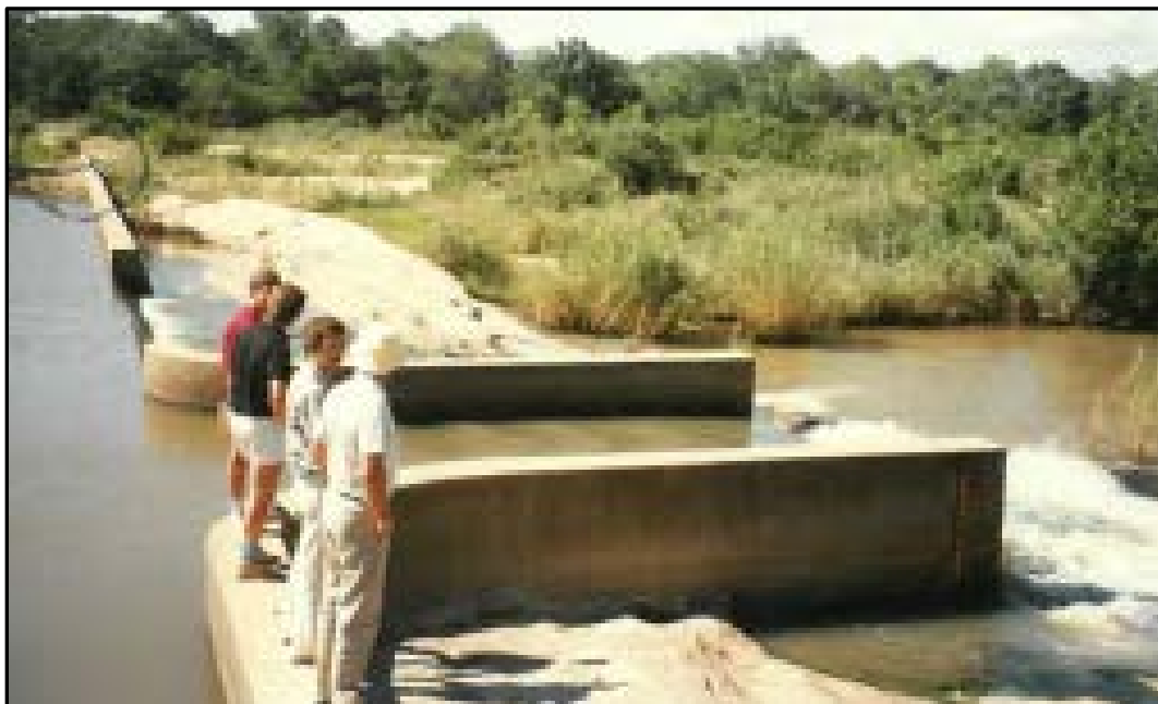
Figure 5.28: Gauging weir X3H008 in the Sand River
