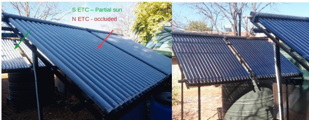
Figure 3.7: a) and b) ETC panels. Note main reservoir in rear, right, Fig 3.7b.
