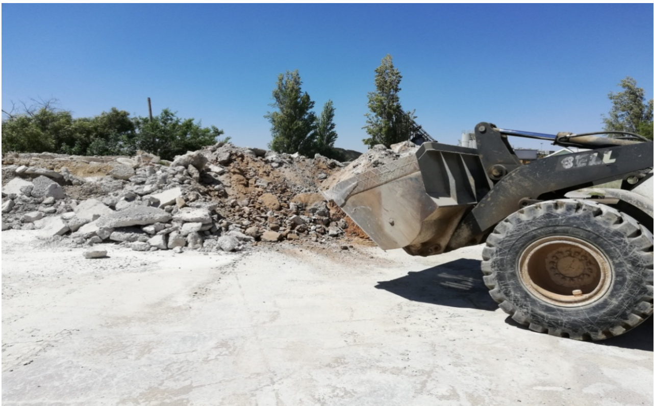
Figure 4.1 Returned readymix concrete rubble used in this study
