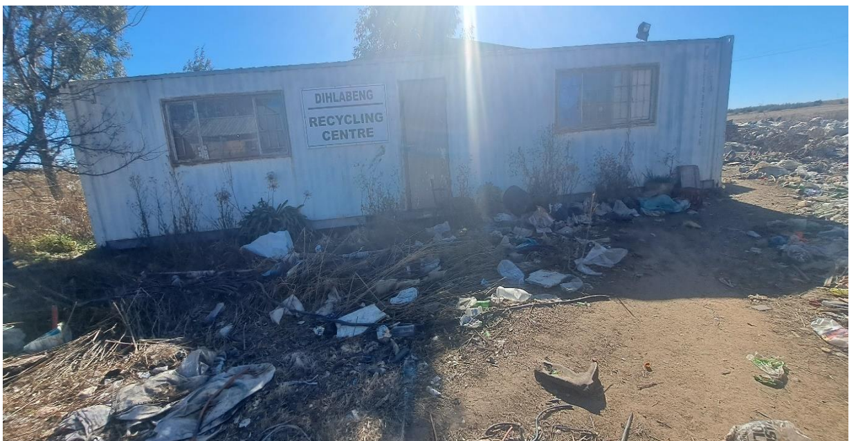
Figure 4.28: Dihlabeng LM: Dilapidated waste recycling centre (© Lepheana: 14/06/2023).
