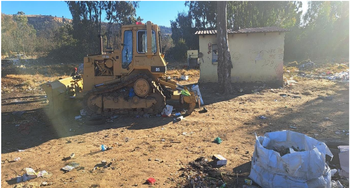
Figure 4.23: Setsoto LM: Waste processing equipment on-site (© Lepheana: 14/06/2023)
