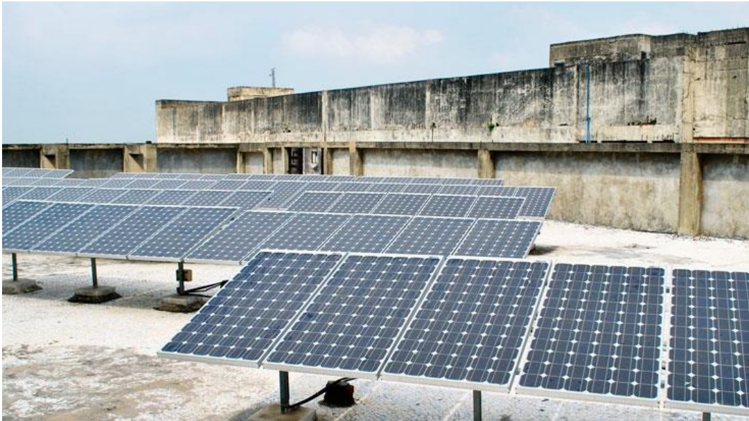
Figure 2.7: PVs installed on flat roof: BAPV type
